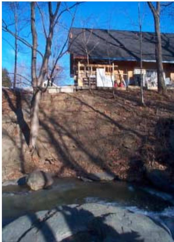
A view of the right bank of the Stevens Brook along the reach between Lincoln Ave. and Barlow St. The stormwater runoff from this residential property flows over the bank causing streambank erosion.
