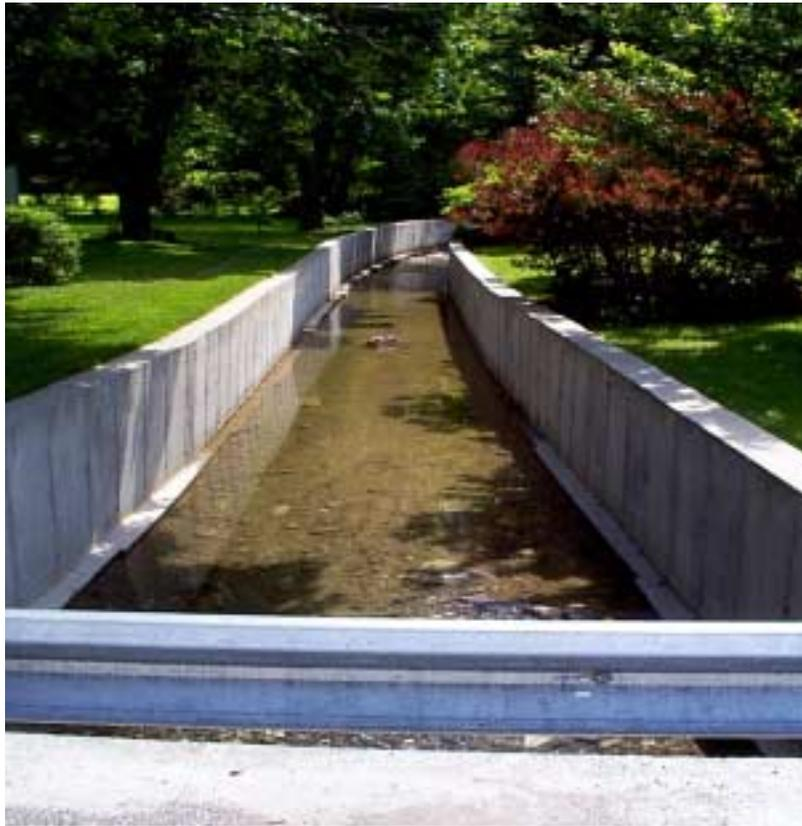
Looking upstream from Quinton Court at the channelization of the stream. This structure concentrates discharge velocities in the stream, which impacts the stream channel downstream.
